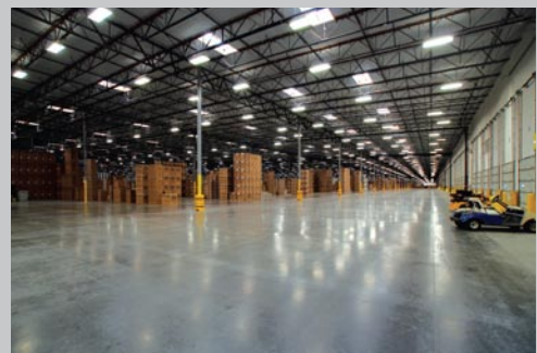
Skylights are the primary source of illumination, with lamps switching on as a secondary option.
