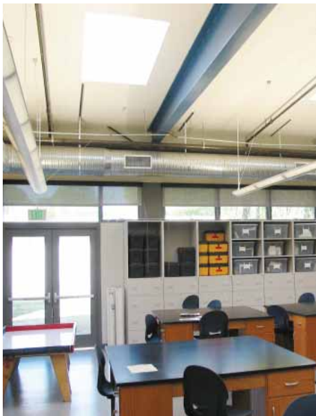
Top-lit applications present a straightforward daylight harvesting control strategy
